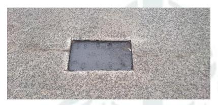
If primers are not to be used the area should be SSD (Saturated Surface Dry) prior to application to prevent suction of water from the HIGHSEAL PR. Ensure not surface water.
